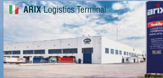
ARIX Logistics Terminal Piattaforma Distributiva - Logistics Terminal Total Area: 48.000 mq - Buildings: 10.200 mq
